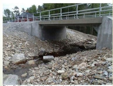
Picture 1b. Object 191 after, bridge with a natural riverbed.
