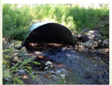
Picture 2b. Object 44 after, arch with natural riverbed.
