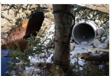
Picture 3b. Otter mitigation, a dry culvert for otters to go through, object 197.
