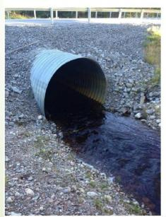
Picture 4b. Object 59, after, a culvert which is lowered and increased culvert to let the riverbed continue under the road
